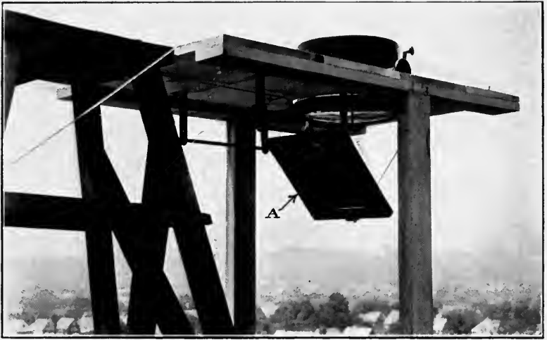
When used as a Landing Light on an Airplane, the Convex-Mirror A was lowered as shown and the beam directed to any spot on the Landing Field
